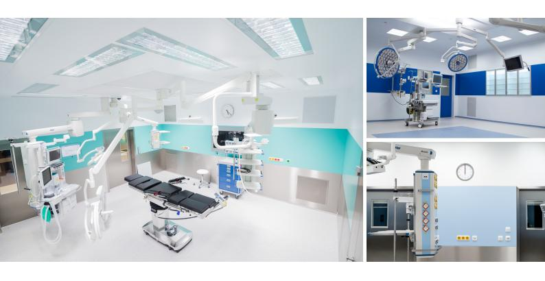
Basic Surgical panels form the final surface of the entire partition system. The system is divided horizontally into three parts.
