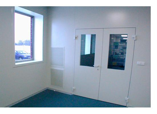
It is inserted into the existing partition panels, thickness 60, 80, 100 and 120 mm.
