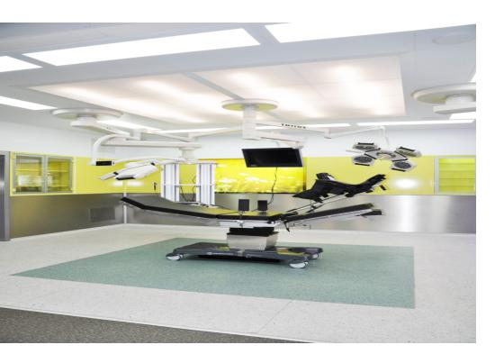
The code is used to specify suspended ceiling panels of atypical dimensions. Ceiling panels of hue RAL 9016 and 9002 are made of painted galvanized steel sheet, thickness 0.6 mm. Panels of other RAL hues are made of galvanized steel sheet, thickness 0.6 mm, surface-finished with thermosetting powder
