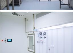
Circulating units are used to supply filtered air to a workplace and to protect the product from ambient contamination. The circulating unit is to be installed in clean rooms of all purity classes. When installing the circulating unit in areas without a defined purity class or in an environment with increased dust generation, a pre-filter is mounted at its suction inlet.
