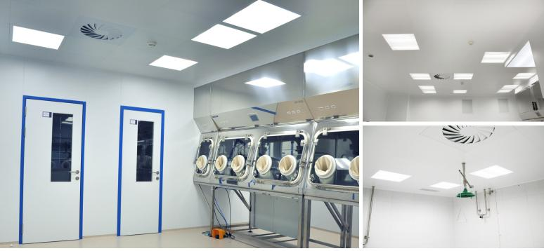
Fluorescent lamps For Clean Light are used for the lighting of interiors with a controlled class of cleanliness. They are mounted into the lightweight metal suspended ceiling FOR CLEAN, they are air-tight, thereby ensuring pressure tightness of the entire suspended ceiling. The light fixture features IP 54 ingress protection according to EN 60529 (IEC 529).
