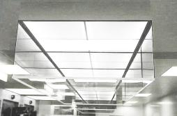
Laminar fields are used to direct incoming air from PUROFIL filtration adapters.
