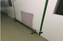
Air conditioning grilles with pocket filters are used to exhaust air from rooms or from locations with dust generation. They prevent the transmission of pollutants and dust particles to the exhaust system. When exhausting air to air ducts from clean partitions, it is sufficient to fit the opening in the partition with a frame featuring a grille and a pocket filter.
