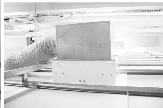
PUROFIL terminal diffusers are intended as an end filtration element in the air distribution system for environments with high demands for the purity of incoming air - such as operating theatres, sterilisation rooms, intensive care units, different areas in pharmaceutical industry, electrical engineering industry, mechanical engineering industry, food industry, etc.
