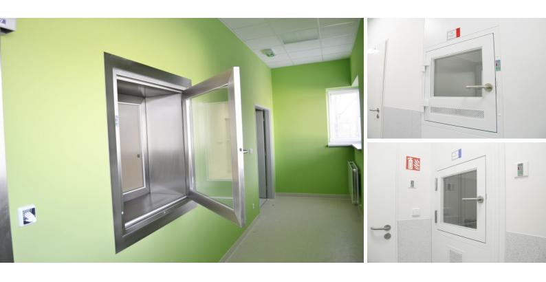
This glazed revolving door is intended for use in clean areas as a material pass-through. It is used to transfer materials between rooms with different classes of cleanliness.
