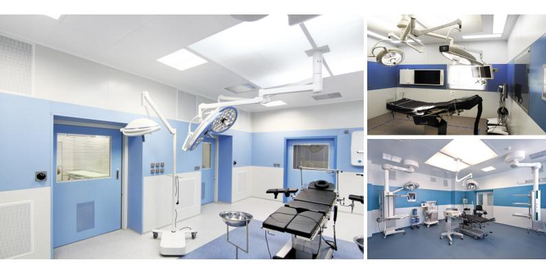
The laminar flow field for operating room are used to create a uniform airflow of specific cleanliness in septic and aseptic operating theatres.
