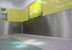
Basic Surgical panels form the final surface of the entire partition system. The system is divided horizontally into three parts.
